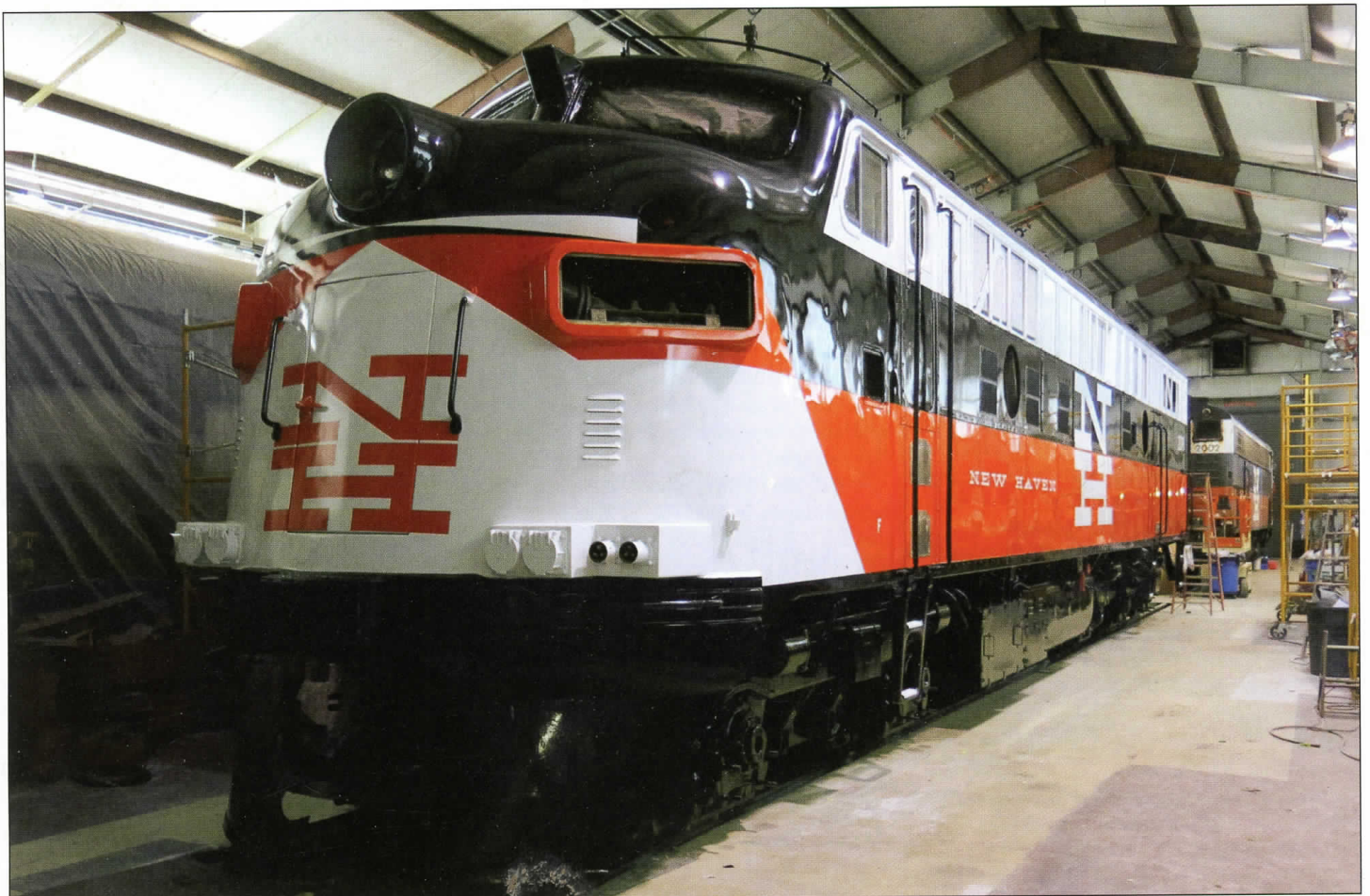
The #2019 is seen freshly painted. Grills, letterboards, etc. await installation. Photo by Bill Sample.
