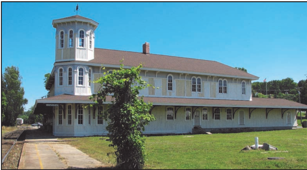
The final phase of the renovation and rebuilding of Canaan Union Station has begun with extensive work on the interior spaces left to complete. The fully realized restoration is slated to include a restaurant, offices and railroad museum.
