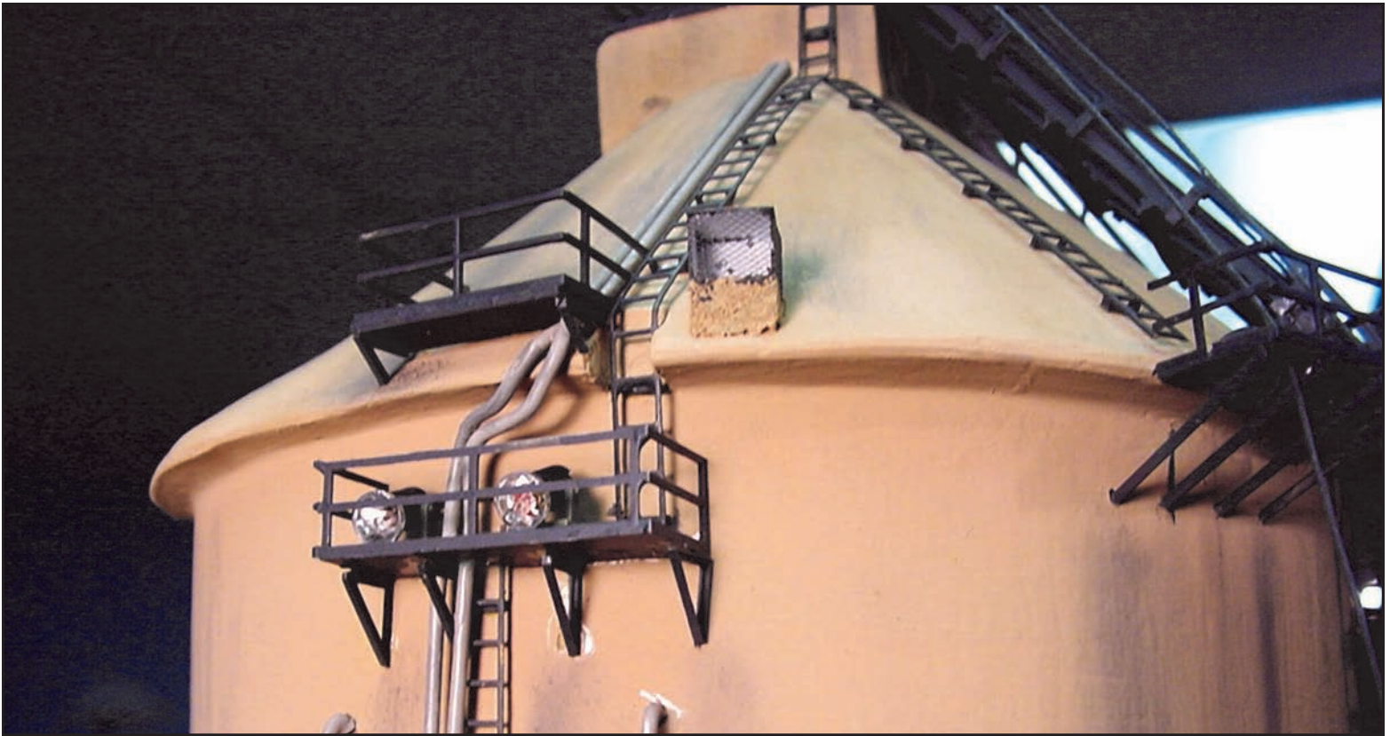
Above: Detail view of tower's floodlights, bunker ventilation duct and sand delivery piping.
