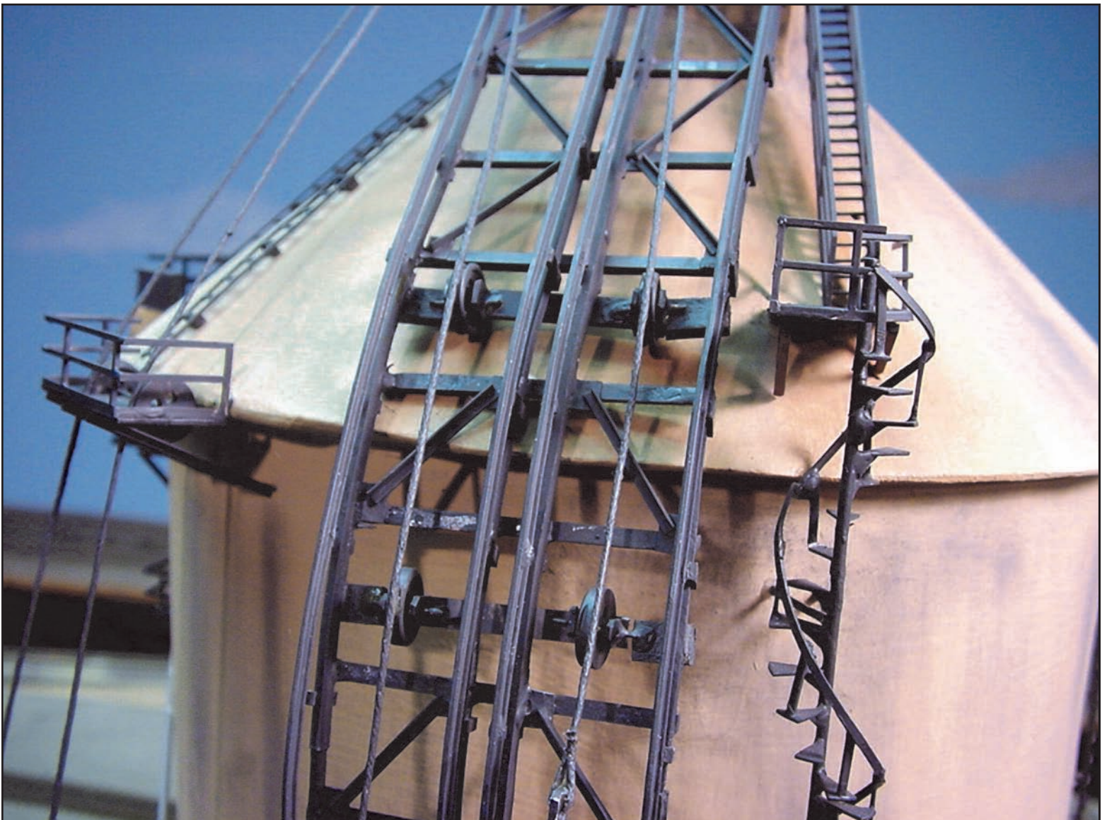
Above and Below: Hoist and coal loading trackway at the top of the tower and curving down the face of the bunker. Note the hoist cables to the left in each photo leading down to the Hoist House. Photos: Lee Ritchie
