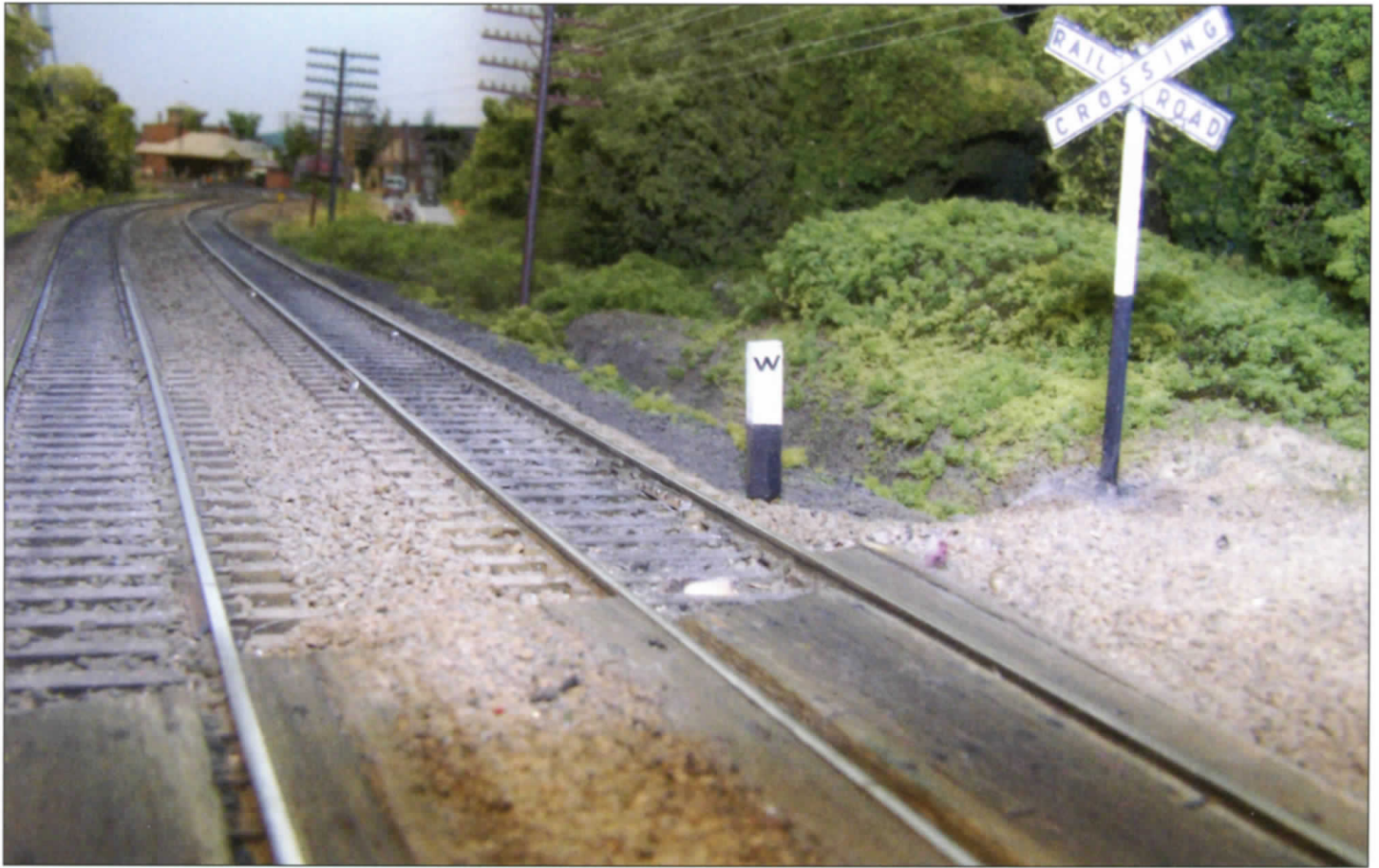
Above: RAILROAD CROSSING DETAILS whistle post for grade crossing not visible beyond the curve and cross bucks guarding the crossing in the foreground. Note the planked crossing on the rural dirt road. Left: This view is from the other side of the crossing above. FLANGER SIGN for grade crossing in the distance. Below: RULE 26 BLUE FLAG POST was blue metal flag and post. In 1947 "RULE 26" was painted on the flag.
